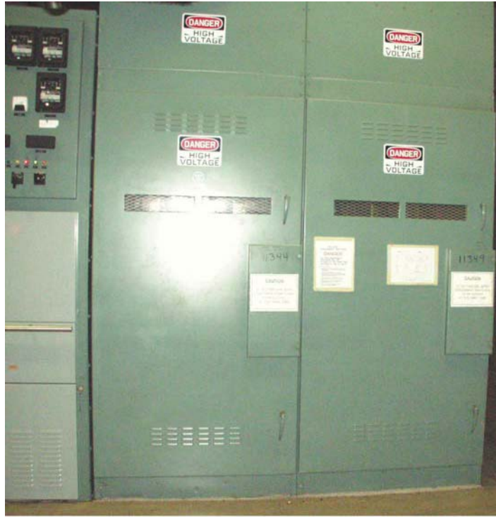
Fig. 1 WESTINGHOUSE 34.5KV LOAD INTERRUPTER SWITCH TYPE WLI
