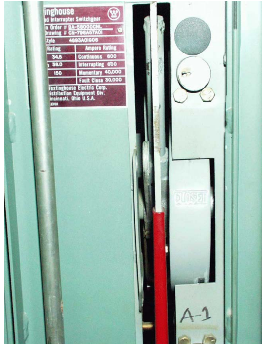
Fig. 3B WLI SWITCH IN CLOSED POSITION ( with removable slow close handle on the left)
